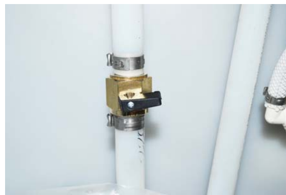
Water Tank Drain Valve -Typical installation shown
