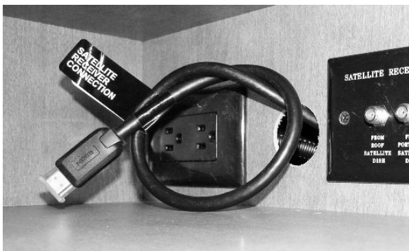
HDMI Cable (Located in front overhead cabinet) -Typical View
