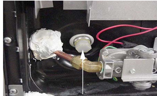
Water Heater Drain Plug (Remove with socket)
