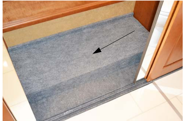
Access Panel (Located on bathroom wardrobe floor)
