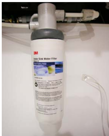
Galley Cold Water Faucet/Ice Maker Filter Assembly (Located below galley sink)
