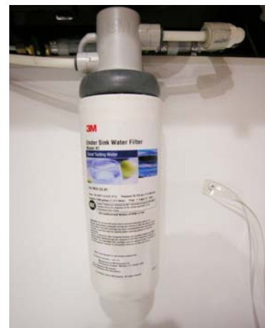
Cold Water Filter Assembly (Located below galley sink) NOTE: Hot waterline is not filtered.
