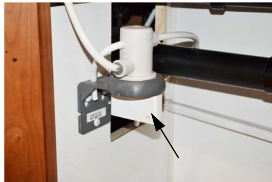
Diverter Plug (installed in filter socket)
