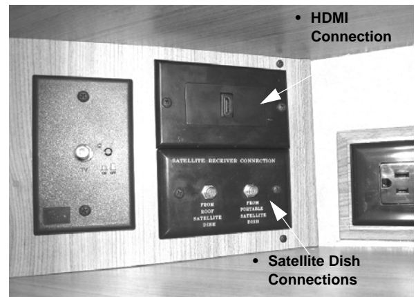
Interior Satellite Dish and HDMI Connections (Located in an overhead cabinet or mounted on a wall near the TV) -Typical installation shown
