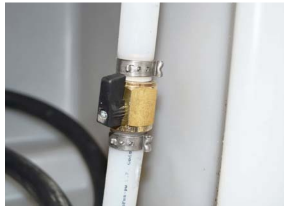
Water Tank Drain Valve -Typical installation shown
