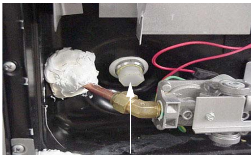
Water Heater Drain Plug (Remove with socket)
