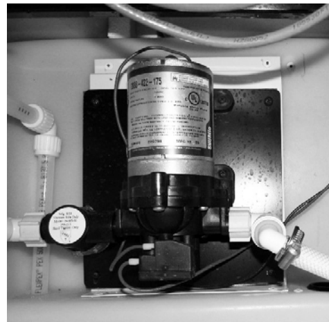
Water Pump -Typical installation shown
