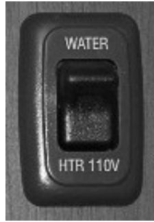
Electric Water Heater Switch (Located near monitor panel)
