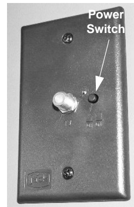
TV Signal Amplifier Power Switch (Located near entertainment center cabinet) -Typical View
