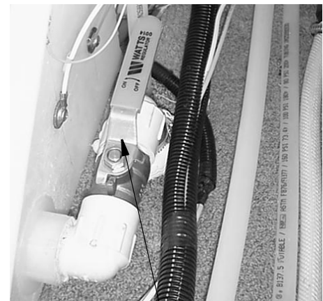
Water Tank Drain Valve -Typical Installation
