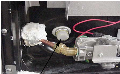
Water Heater Drain Plug (Remove with socket)
