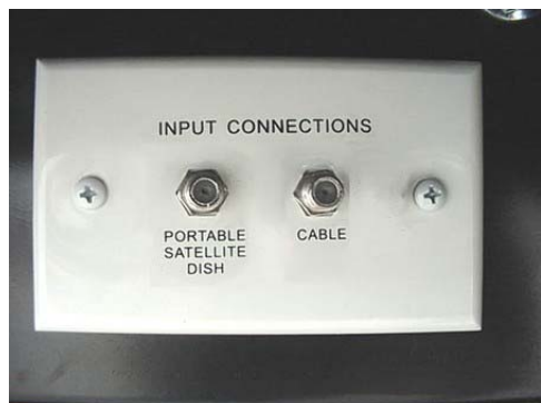
Satellite Dish and Cable TV Connections (Located in utility compartment or water service center) -Typical View
