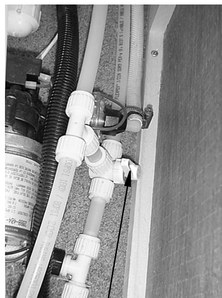
Waterline Drain Valve (Typical)
