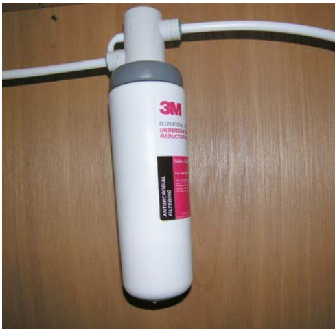
Cold Water Filter Assembly (Located below galley sink) NOTE: Hot waterline is not filtered
