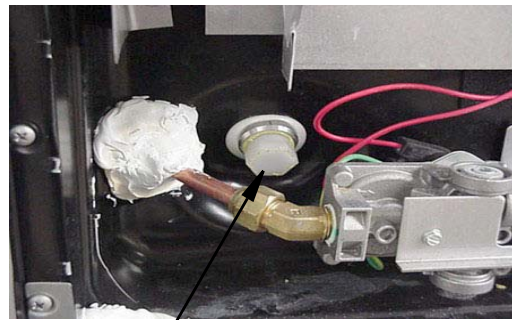
Water Heater Drain Plug (Remove with socket)
