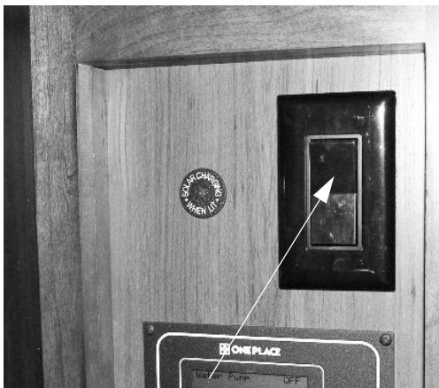
Diesel Engine Heater Switch (Located near monitor panel) -Typical View
