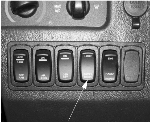
Power Door Locks - Entry Door (Located on dash) -Typical View
