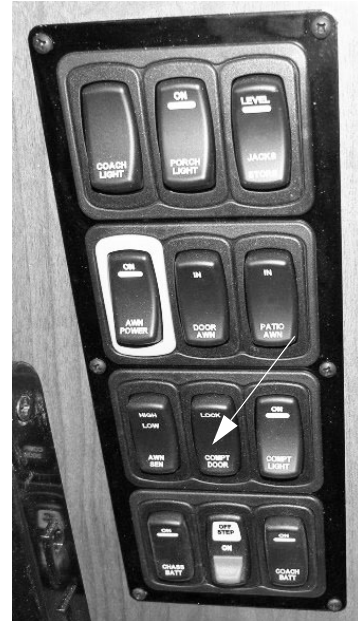
Power Door Locks - Compartment Doors (Located on entry switch panel) -Typical View
