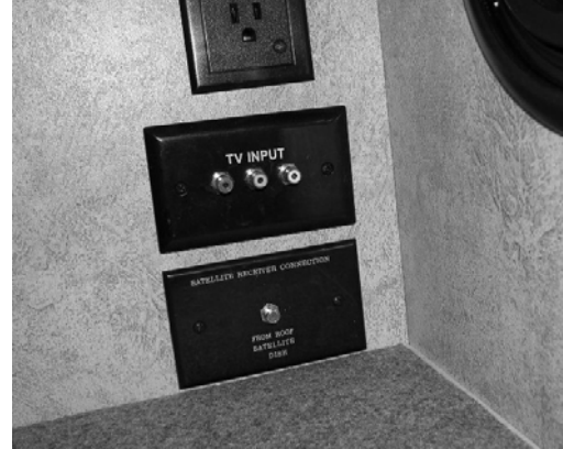
Bedroom DVD/Satellite Receiver Connection -Typical View
