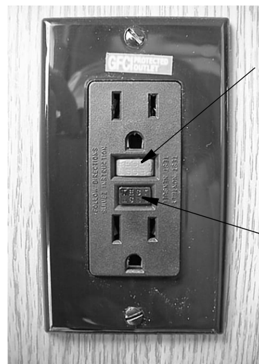
GFCI Outlet (Ground Fault Protector)
