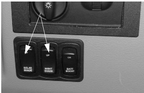
12-Volt Front Drop-Down Solar/ Night Shade Switches (Located on dash) -Typical View
