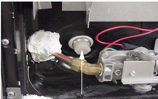
Water Heater Drain Plug (Remove with socket)
