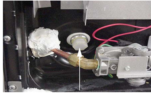
Water Heater Drain Plug (Remove with socket)
