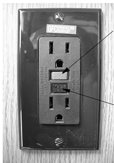
GFCI Outlet (Ground Fault Protector)
