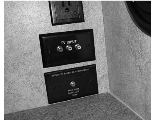
Bedroom DVD/Satellite Receiver Connection -Typical View
