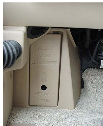
Automotive Fuse/Breaker Panel (Located beneath left end of dash)
