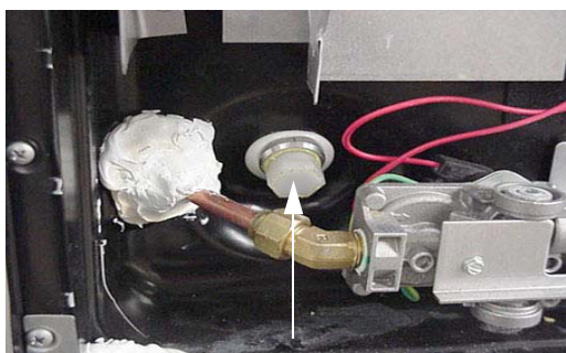
Water Heater Drain Plug (Remove with socket)
