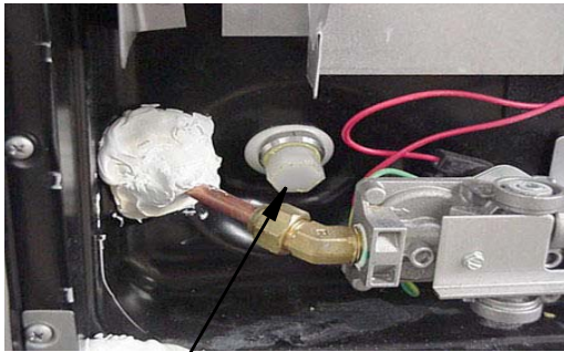
Water Heater Drain Plug (Remove with socket)
