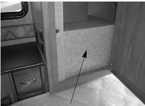
Water Heater Bypass Valve Access (Located within wardrobe - remove front panel to access)
