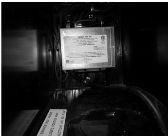
Automatic Power Transfer Box (Located inside utility compartment)
