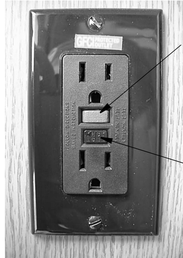
GFCI Outlet (Ground Fault Protector)
