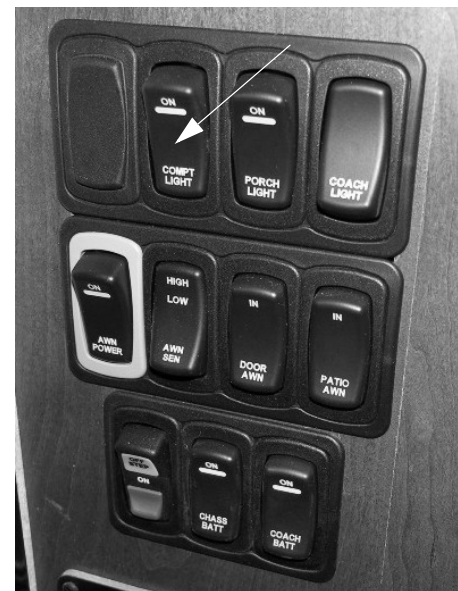
Compartment Lights Switch (Located near entrance door) -Typical View
