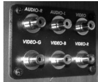
Audio Video Connection Plate -Typical View
