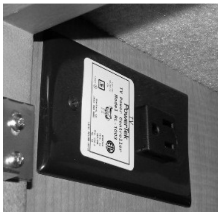
Front TV Ignition Switch Interlock -Typical View
