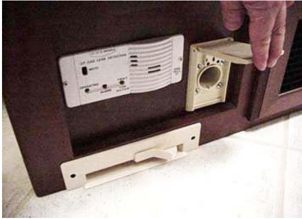
Central Vacuum Cleaner System -Typical View
