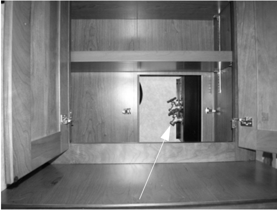
Water Supply Faucets -Typical Installation
