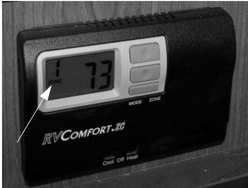
Zone 1 Operation (Living Area/Galley)
