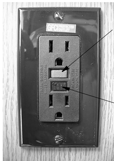
GFCI Outlet (Ground Fault Protector)
