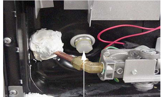
Water Heater Drain Plug (Remove with socket)
