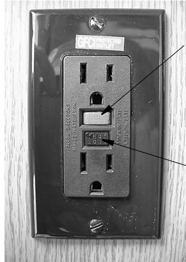
GFCI Outlet (Ground Fault Protector)
