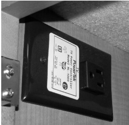
Front TV Ignition Switch Interlock –Typical View
