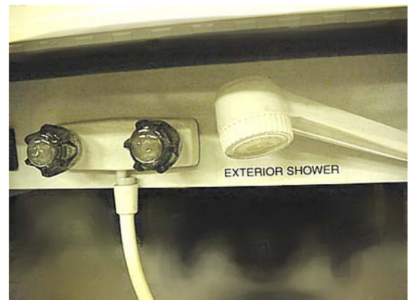
Exterior Shower/Wash Station -Typical View
