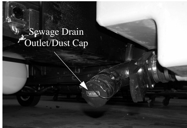
Sewage Drain Outlet/Dust Cap (Located beneath coach on mid-driver side) -Typical View
