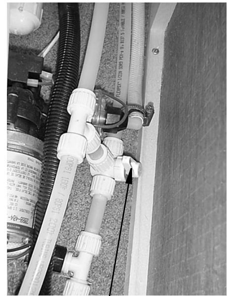
Waterline Drain Valve (Typical)
