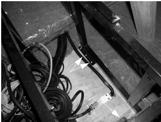
Steel Frame Screw Locations -Typical View
