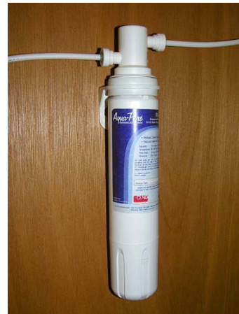
Water Filter Assembly (Located below galley sink)
