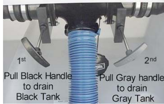
Holding Tank Dump Valves
