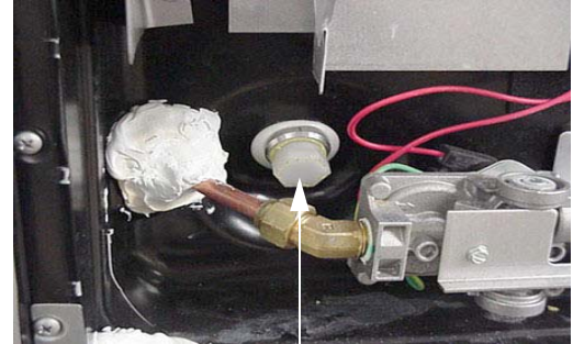
Water Heater Drain Plug (Remove with socket)
