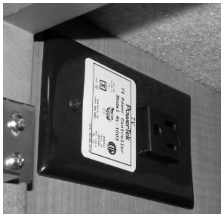
Front TV Ignition Switch Interlock -Typical View
