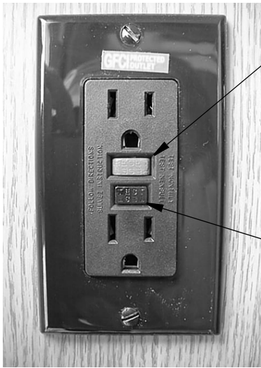
GFCI Outlet (Ground Fault Protector)
