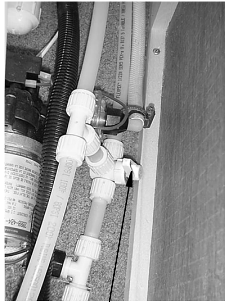
Waterline Drain Valve (Typical)
