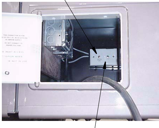
Portable Satellite Dish Hook-up in Shoreline Compartment
