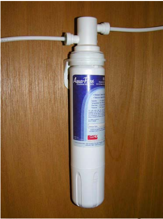
Water Filter Assembly below Galley Sink
