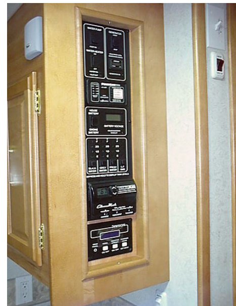
One Place Monitor Panel
