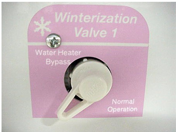
Water Heater By-Pass Valve
