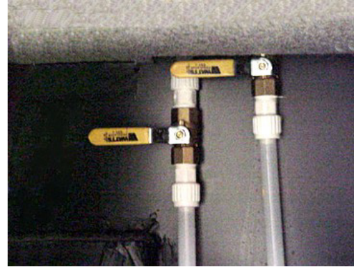
Water Line Drain Valves in Water Center Models 34H & 36G
